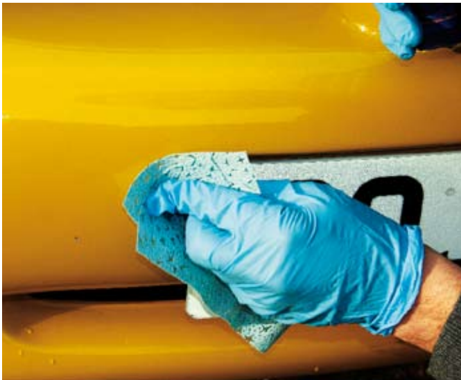
The blending agent then lifts off any excess paint from the panel's surface, leaving the new colour confined within the damaged area.
